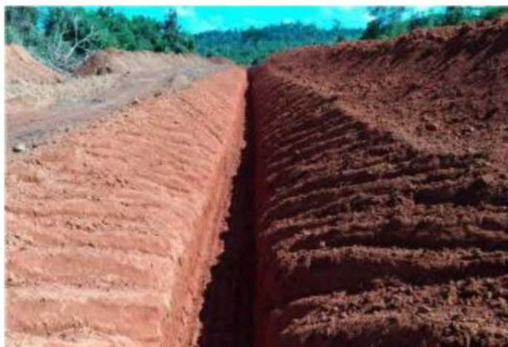
Trenching at the Baldo zone, Cajueiro project
